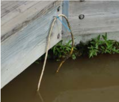
Above: Examples of electrical cords, on the slips, that are not in compliance with the state regulations and will be removed.
